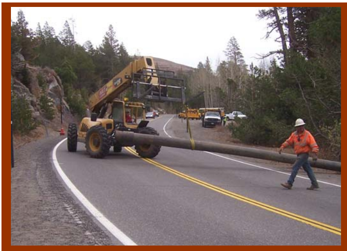
Removing the bypass pipeline
